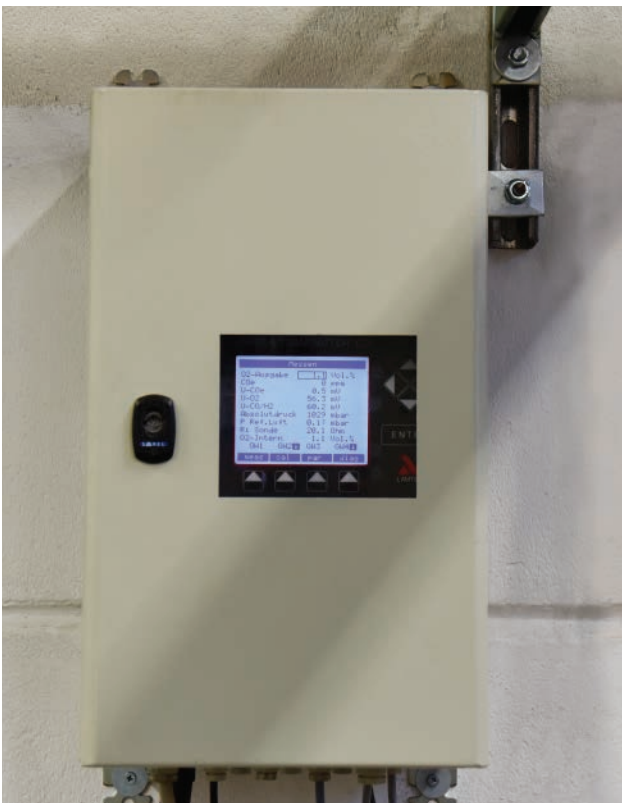
LT2K with integrated reference air pump.
