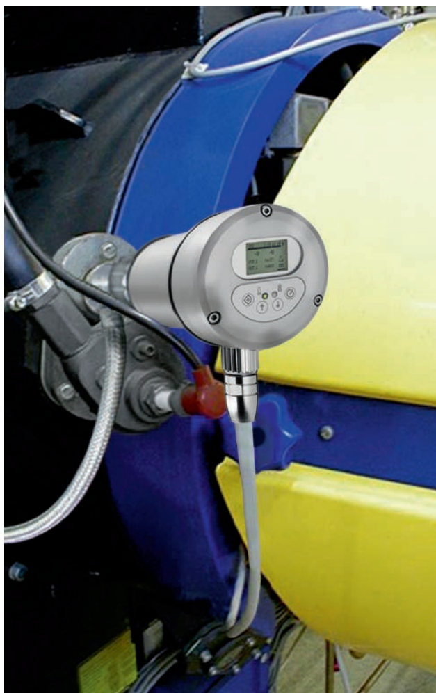
The LAMTEC F300K flame scanner in operation.
